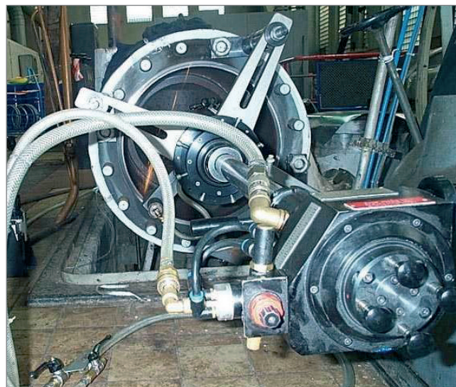
HTS 400 grinding on site
