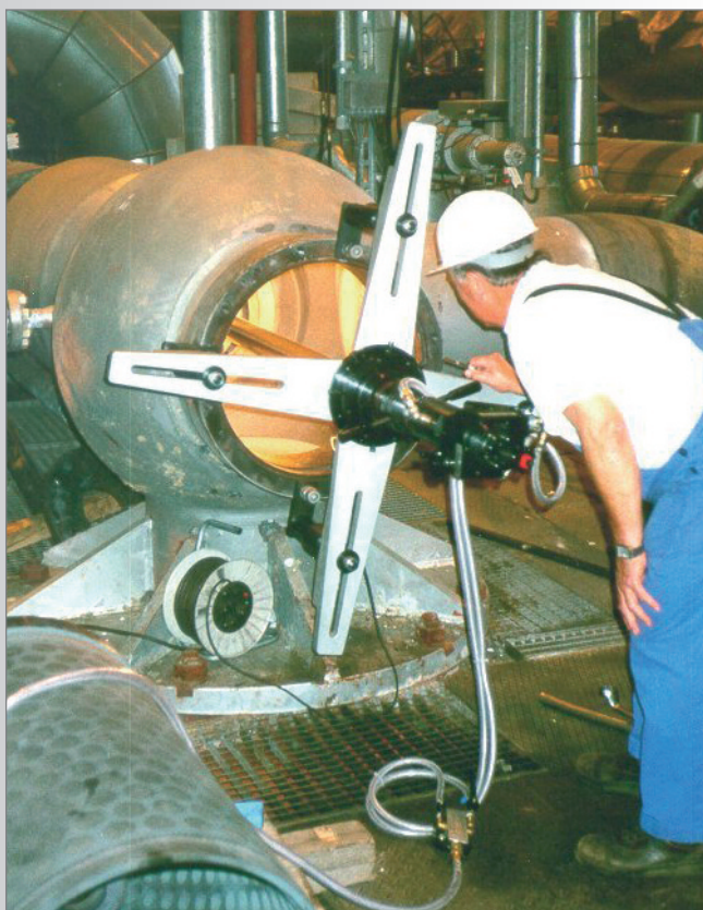
HTS 800 grinding the sealing surface of a Turbine Bypass valve in 1100 mm (44") depth
