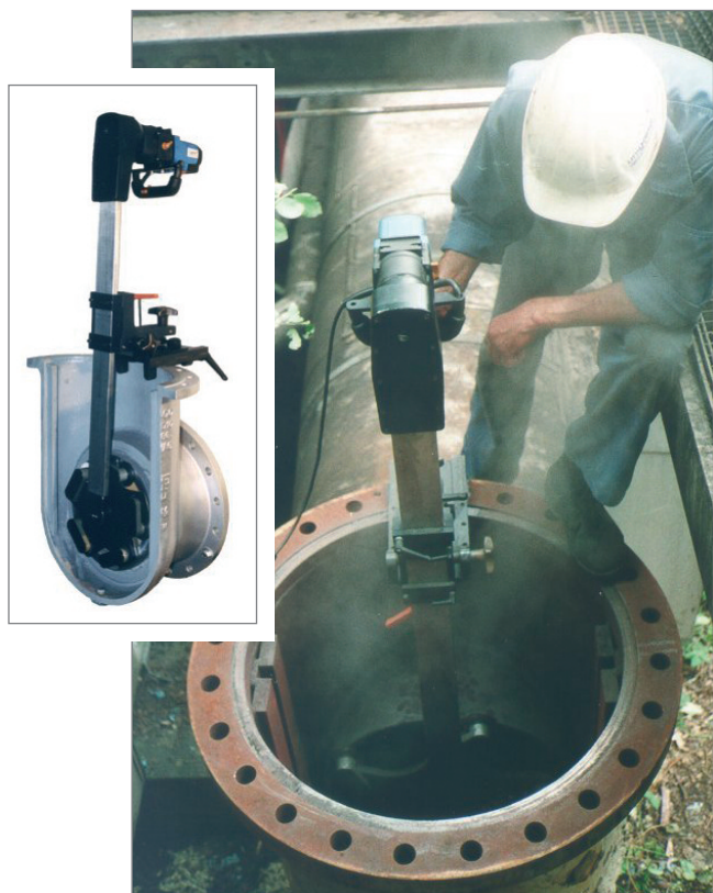
SHS 600 grinding a 24" Gate valve (vertical)
